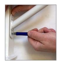
2. Drill the four holes in the cross beam with a 3,5 mm metal drill.
