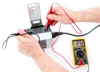
Checking voltage on charger
